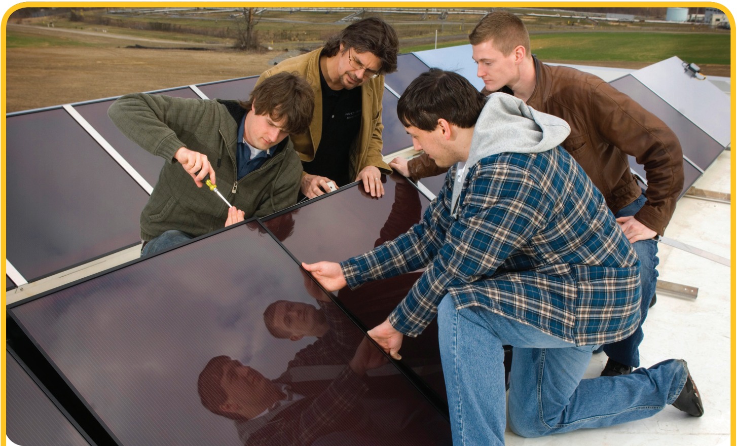
Electrical and computer engineering associate professor Dr. Peter Jansson (second from left) works with students Andy Hak (left), Dane Green (front right) and Ulrich Schwabe to install solar panels on the South Jersey Technology Park's Samuel H. Jones Innovation Center as part of a renewable energy project sponsored by Kaneka, the world's largest manufacturer of thin-film photovoltaic modules. Tenants in the 45,000-square-foot building will include Rowan Engineering, the Rowan Center for Innovation and Entrepreneurship and the Rowan Business Incubator. Space still is available for start-up and established technology businesses in the Technology Park, which is a public-private venture based in Mantua Township, about a mile from Rowan. For more information, visit www.sjtechpark.com .
