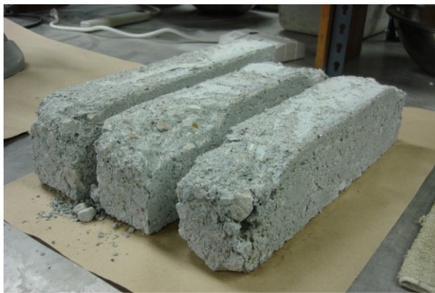
Concrete can deteriorate due to freezing
