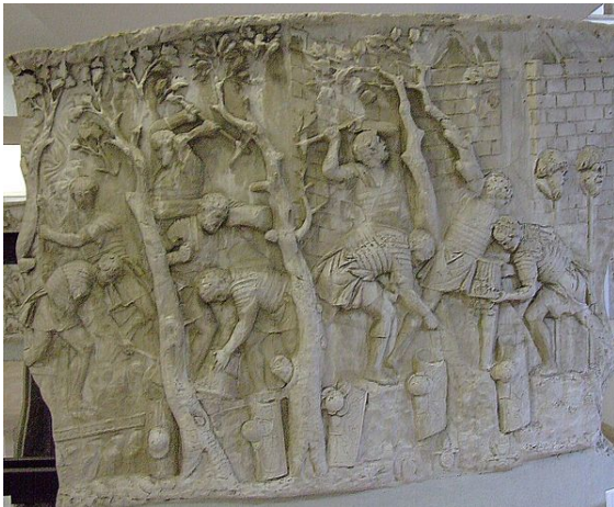
Road construction, depicted on Trajan's Column
