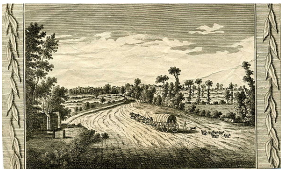
The Great North Road near Highgate on the approach to London before turnpiking. The highway was deeply rutted and spread onto adjoining land.
