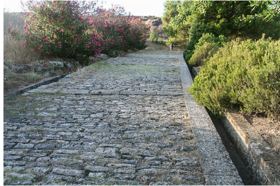
Greek street - 4th or 3rd century BC - The Porta Rosa was the main street of Elea. It connects the northern quarter with the southern quarter. The street is five meters wide and has an incline of 18% in the steepest part. It is paved with limestone blocks and on one side there is a small gutter for drainage.
