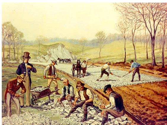
Construction of the first macadamized road in the United States (1823). In the foreground, workers are breaking stones "so as not to exceed 6 ounces in weight or to pass a two-inch ring". [23]
