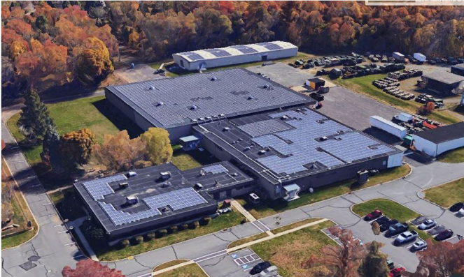
Figure 4. Rooftop solar panel arrays. In FY20, this system generated 464,000 kWh of energy, enough to power 44 typical homes.
